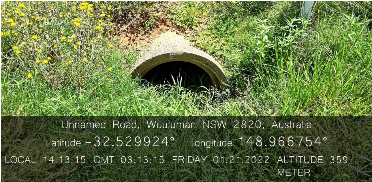
Photograph 6.2 Existing culvert crossing at Watercourse A
